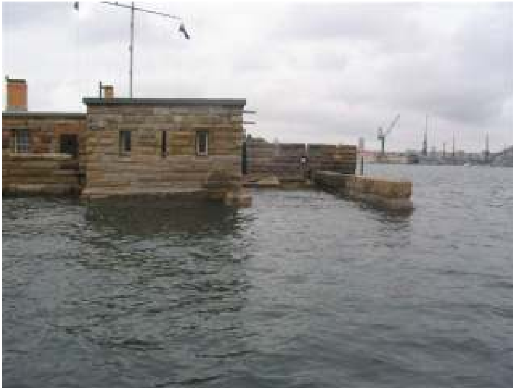
Figure F1: Slipway and West Room at SW end of Fort at 0915 hrs. Measured water level is 1.95m ISLW (1.025m AHD).
