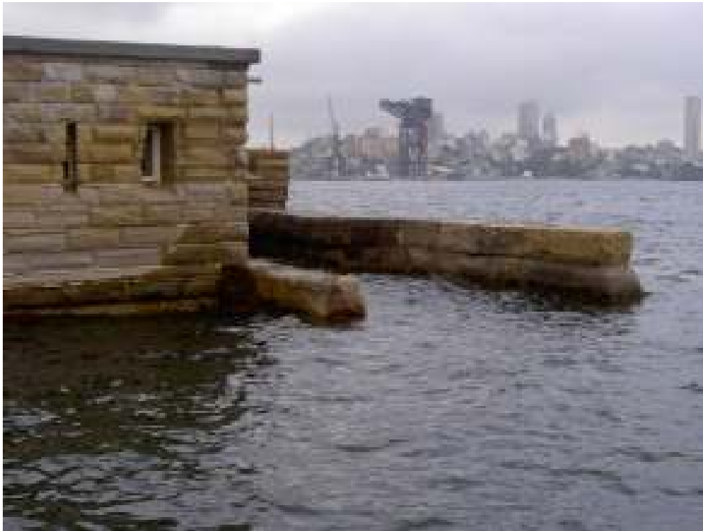
Figure F5: Slipway and West Room at SW end of Fort at 0845 hrs. Measured water level is 1.95m ISLW (1.025m AHD).
