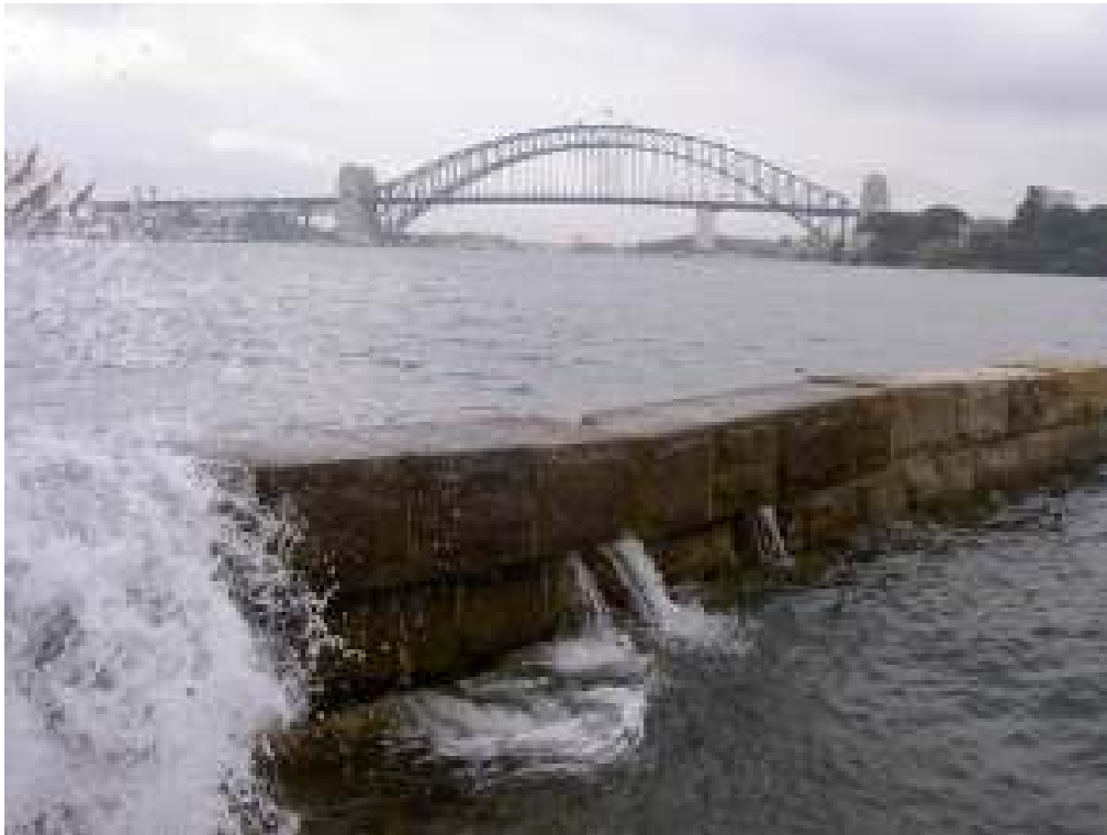
Figure F9: Ferry wave against slipway at SW end of Fort at 0900 hrs. Measured water level is 1.95m ISLW (1.025m AHD).
