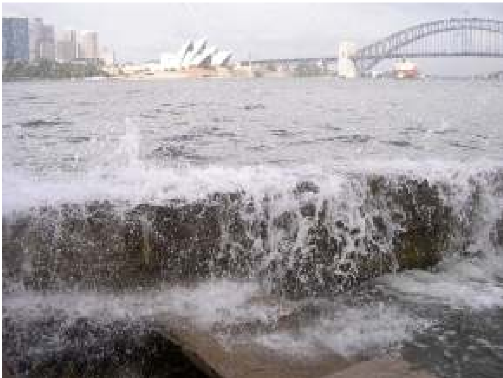
Figure F10: Ferry wave overtopping slipway at SW end of Fort at 0900 hrs. Measured water level is 1.95m ISLW (1.025m AHD).
