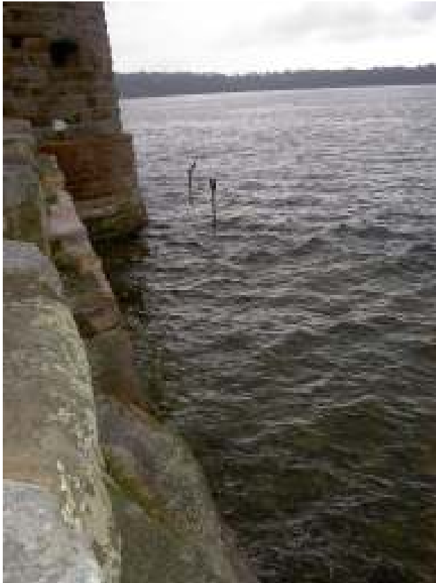
Figure F13: Martello Tower at NE end of Fort at 0915 hrs. Measured water level is 1.95m ISLW (1.025m AHD).
