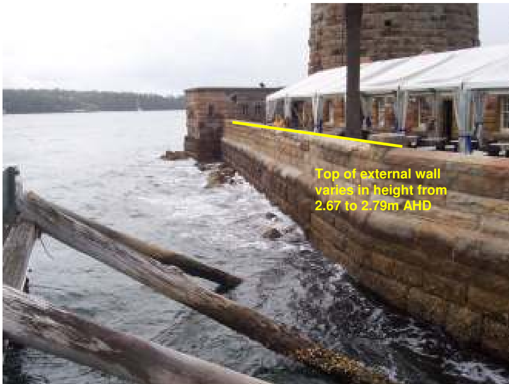
Figure G1: Northern portion of Western Seawall and Tide Room at 1100 hrs on 6 November 2007. Measured water level is 0.53m ISLW (-0.395m AHD).
