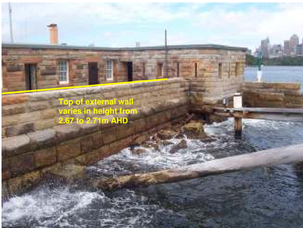
Figure G2: Western Seawall at 1100 hrs on 6 November 2007. Measured water level is 0.53m ISLW (-0.395m AHD).
