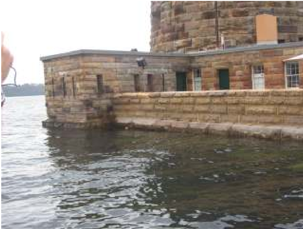
Figure F3: Tide Room and Western Seawall at NE end of Fort at 0915 hrs. Measured water level is 1.95m ISLW (1.025m AHD).
