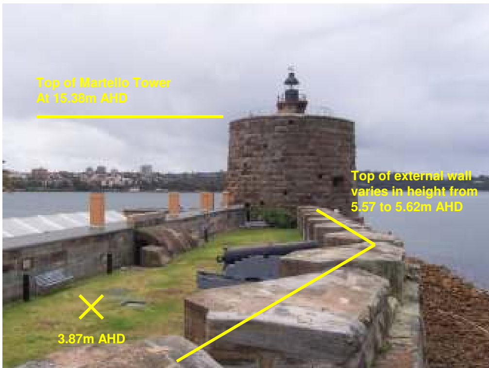
Figure F8: Grassed Eastern Terrace and Eastern Seawall.
